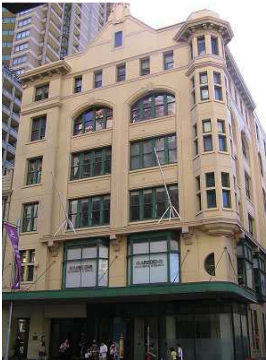
Figure 13 Metters Building. Source: State Heritage Register.
