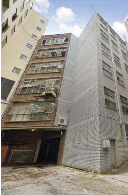
Figure 25 Rear of building – 1970s additions
