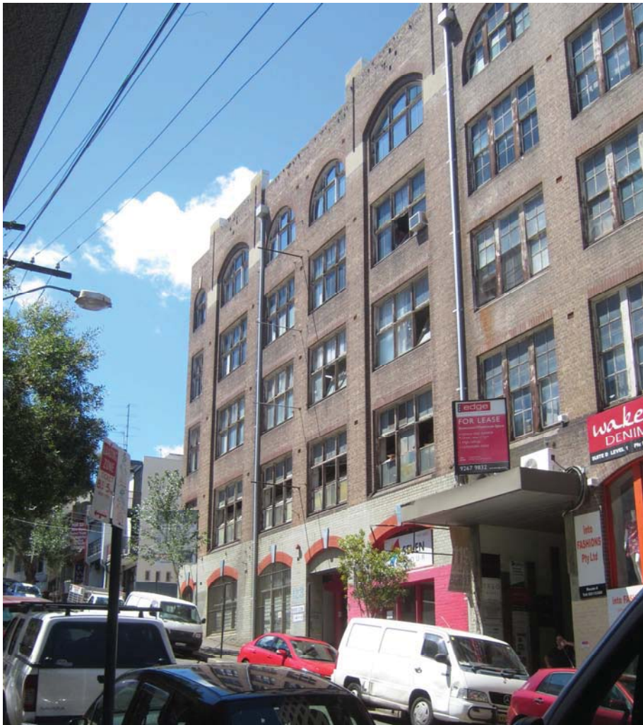
Figure 19 Kippax Street facade.
