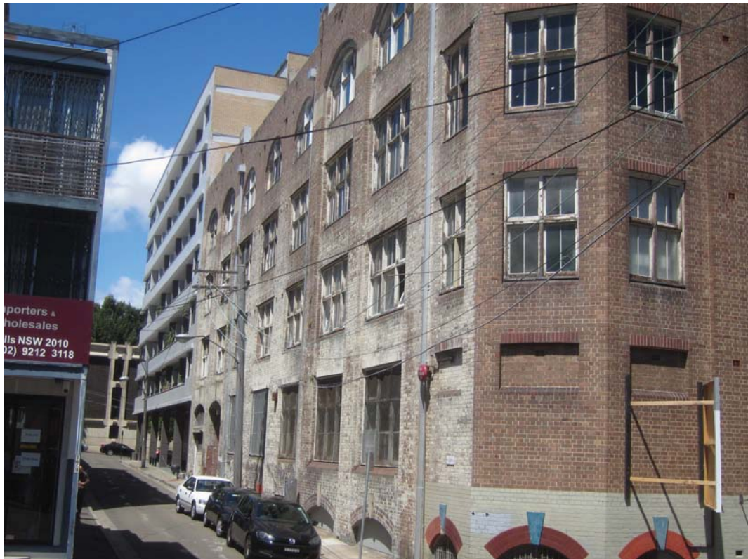
Figure 20 Lacey Street facade
